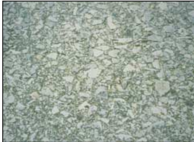
FIGURE 39 Distress Type ACP 12—Polished Aggregate
