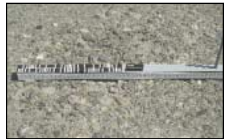
FIGURE 42 Distress Type ACP 13—Loss of Coarse Aggregate
