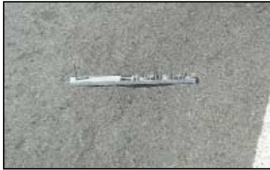
FIGURE 40 Distress Type ACP 13—Loss of Fine Aggregate
